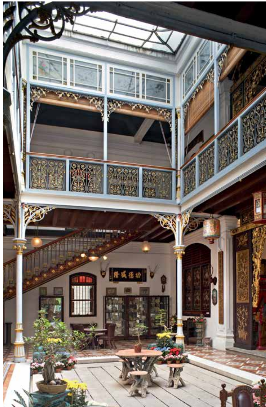
Left: This view looking across the skywell reveals the extravagant use of cast-iron columns, brackets, and balustrades as well as the varying patterns within the adjacent semi-enclosed spaces around the atrium-like space.
